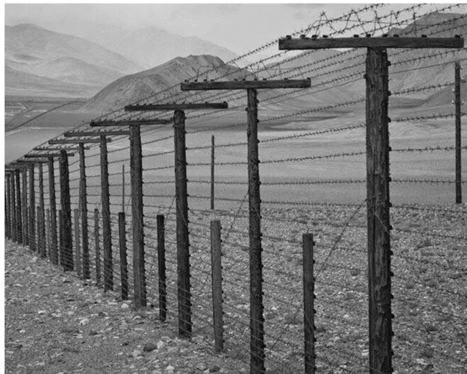
Figure 1 – Security barrier of the S-100 "Skala" alarm system
