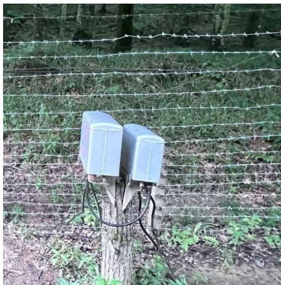
Figure 4 – Linear unit and distribution box of the alarm system S-175 "Gardina"
