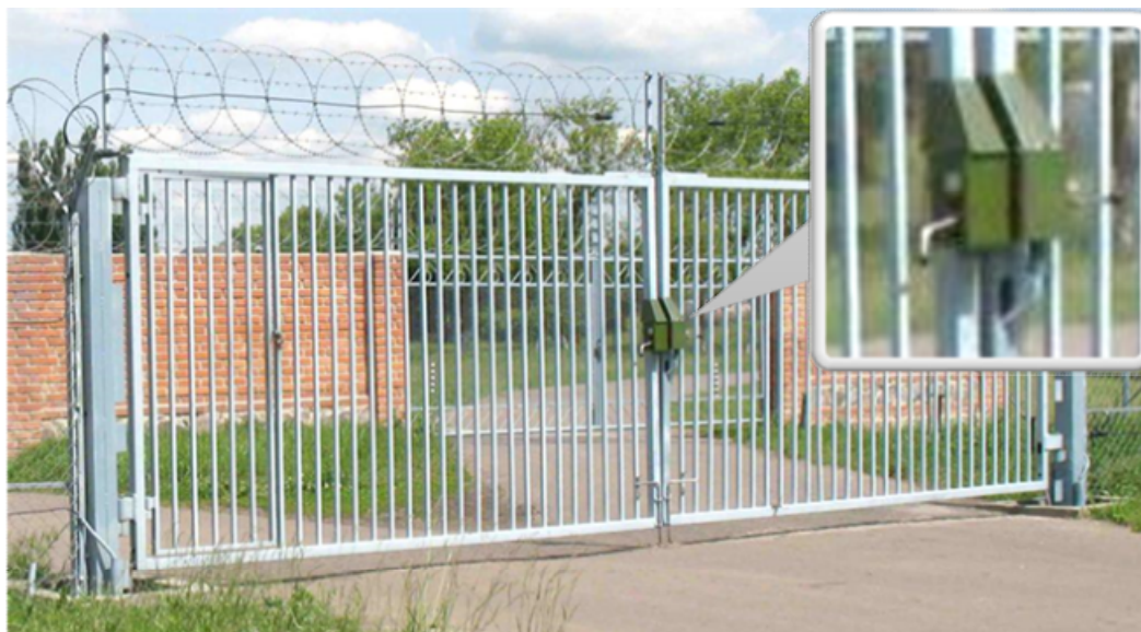
Figure 6 – Locking device on the gate of the linear part of the KS-185 "Gobi" signalling complex
